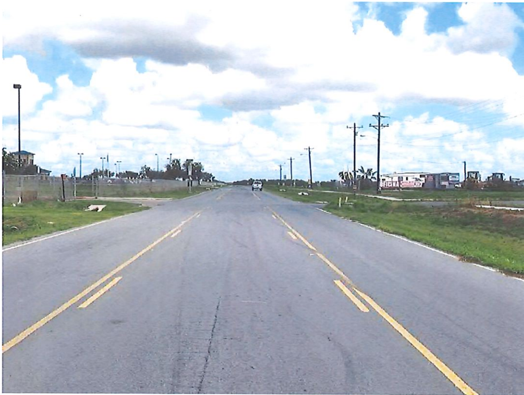
Looking north on Carmen Avila Road, from south of Mile 22.5 North Road
