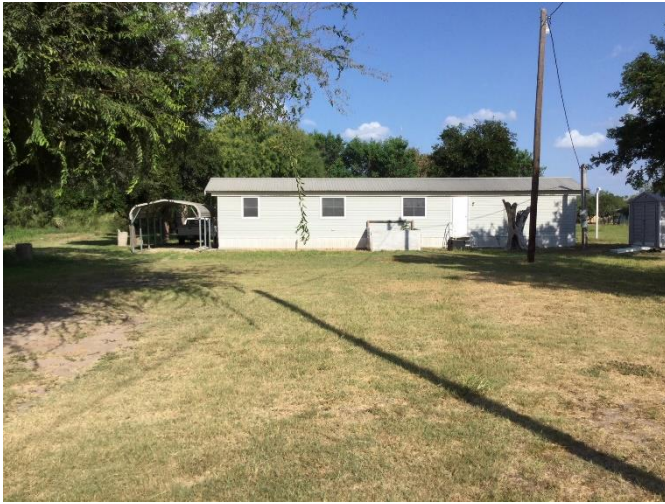
Photo 1 View of subject property
