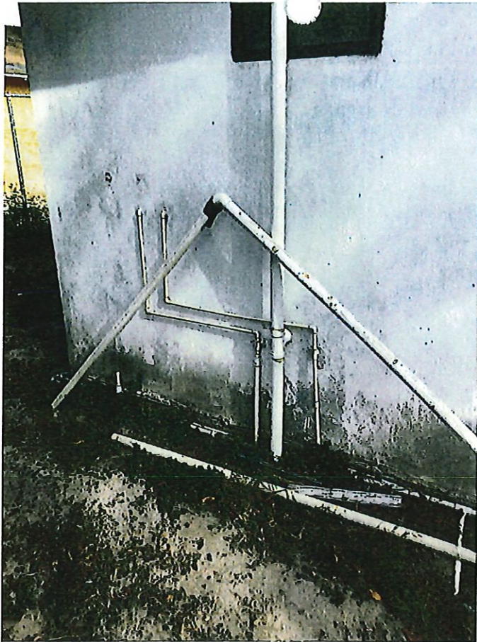
Exposed plumbing Located At rear of House
