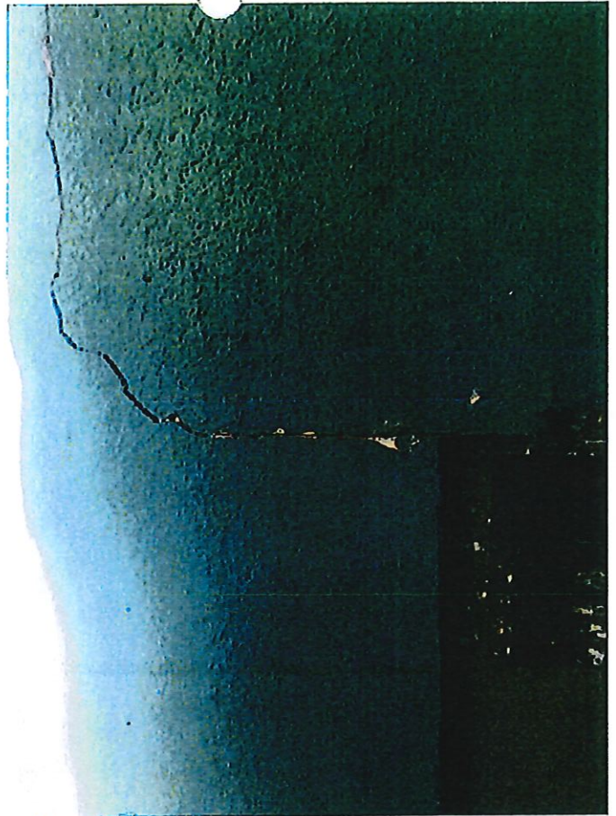
Large crack next to panel box due to foundation movement
