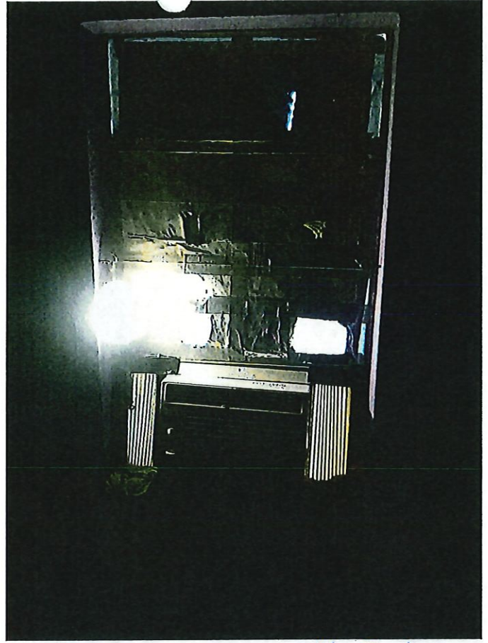
Window in bedroom # 2 does not open. window unit.
