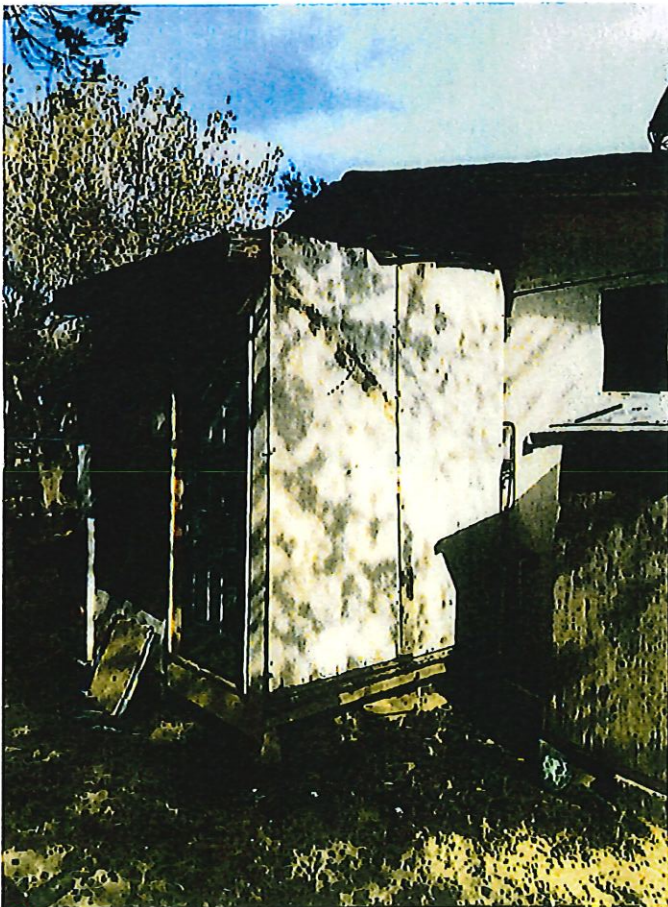
Rear of House "west side" Storage
