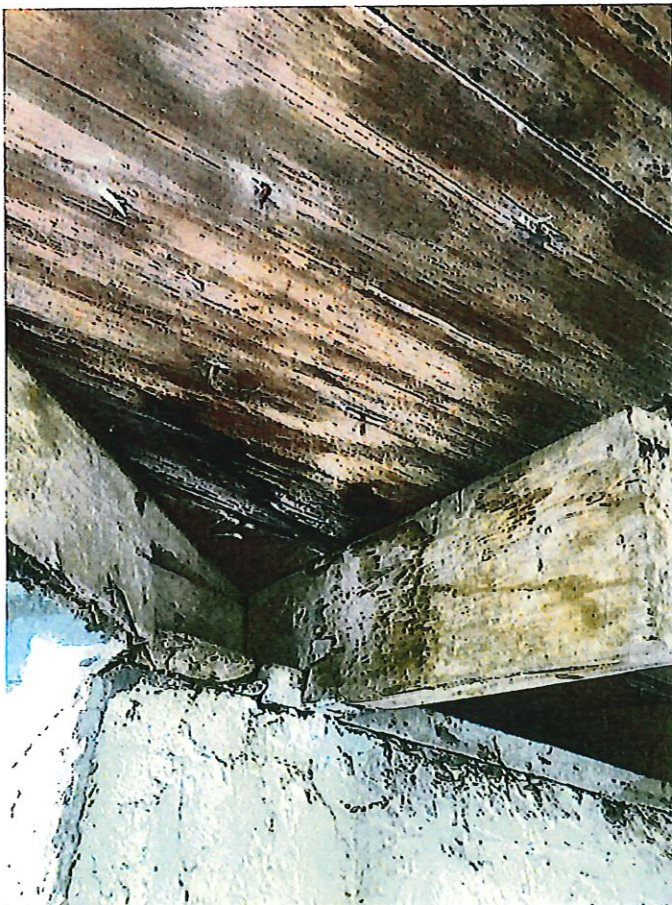
Roof Decking from Carport
