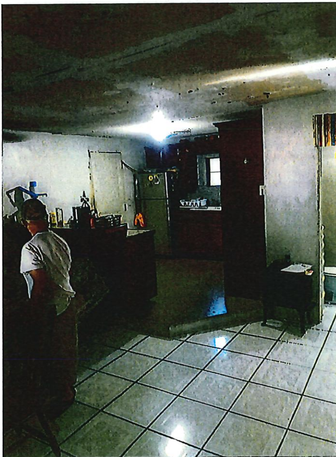
Kitchen view, no paint or texture
