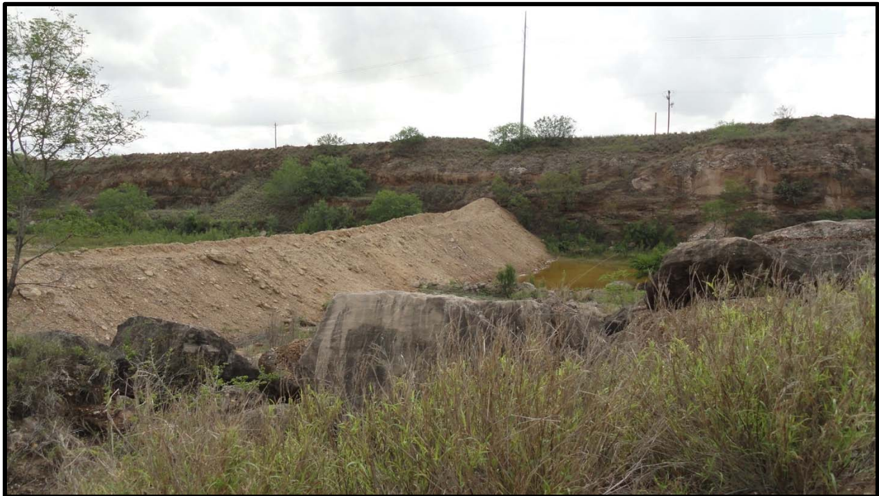
Viewing berm northeast from southeast access road.
