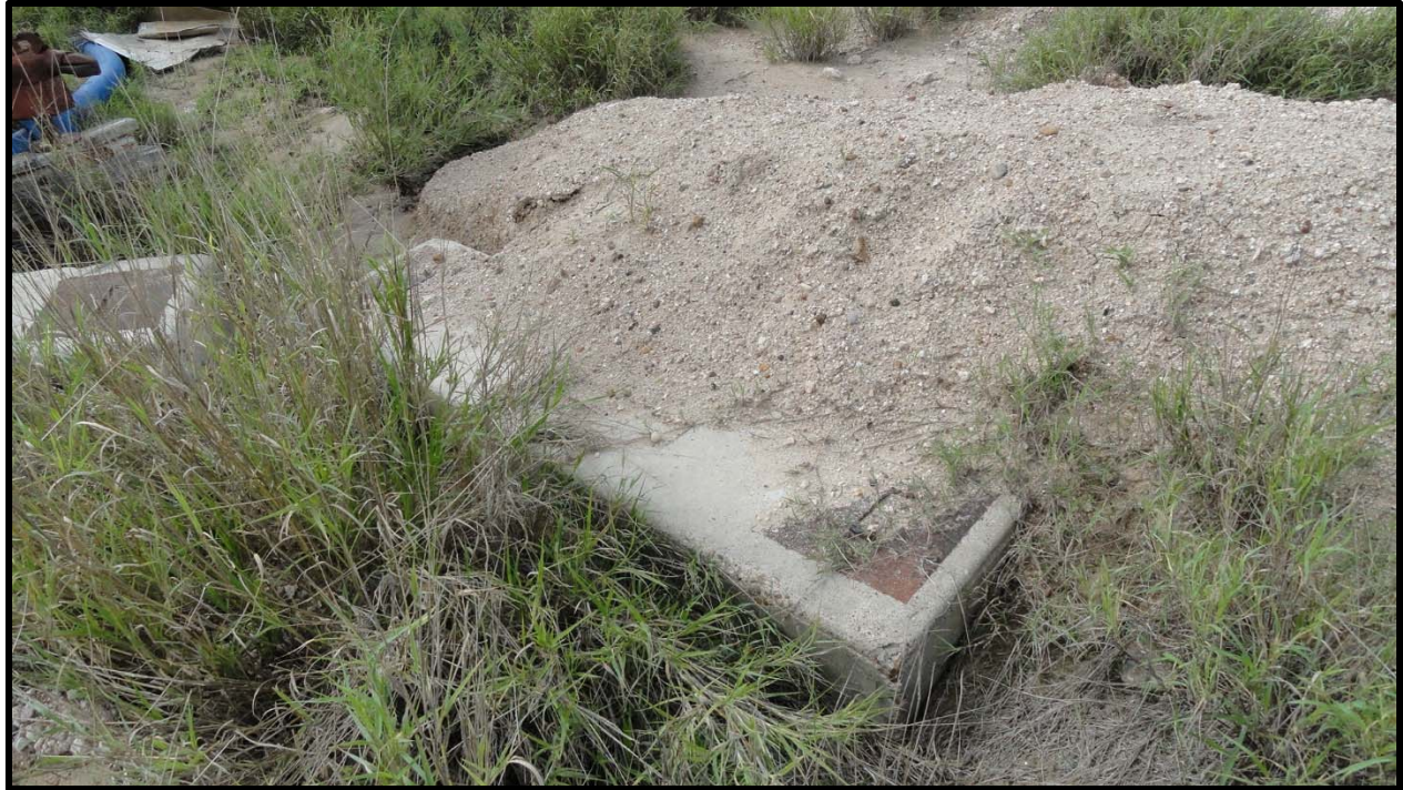
Concrete slabs at the end of the northeast access road.
