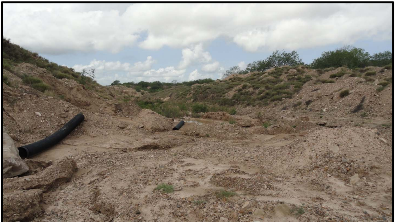
Viewing southwest from southeast access road.
