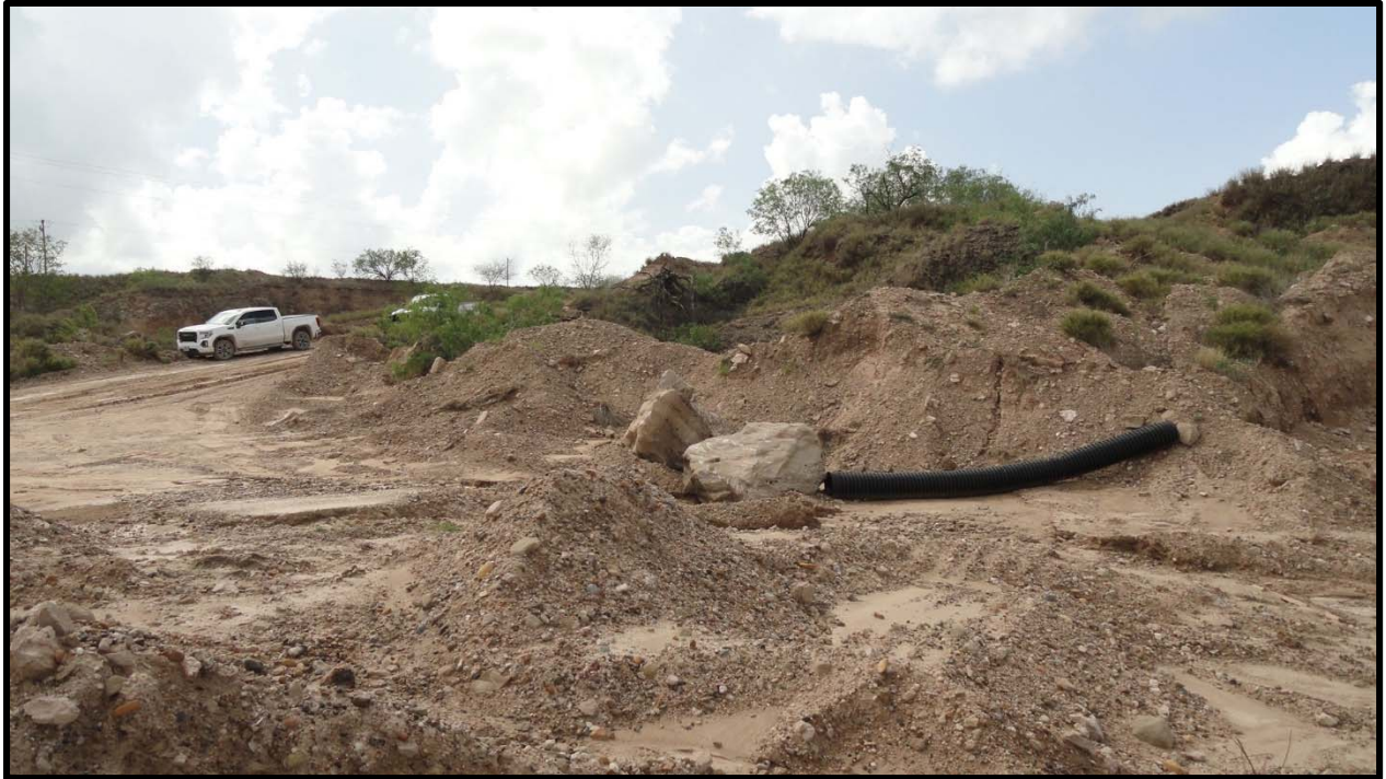
Viewing southeast from southeast access road.
