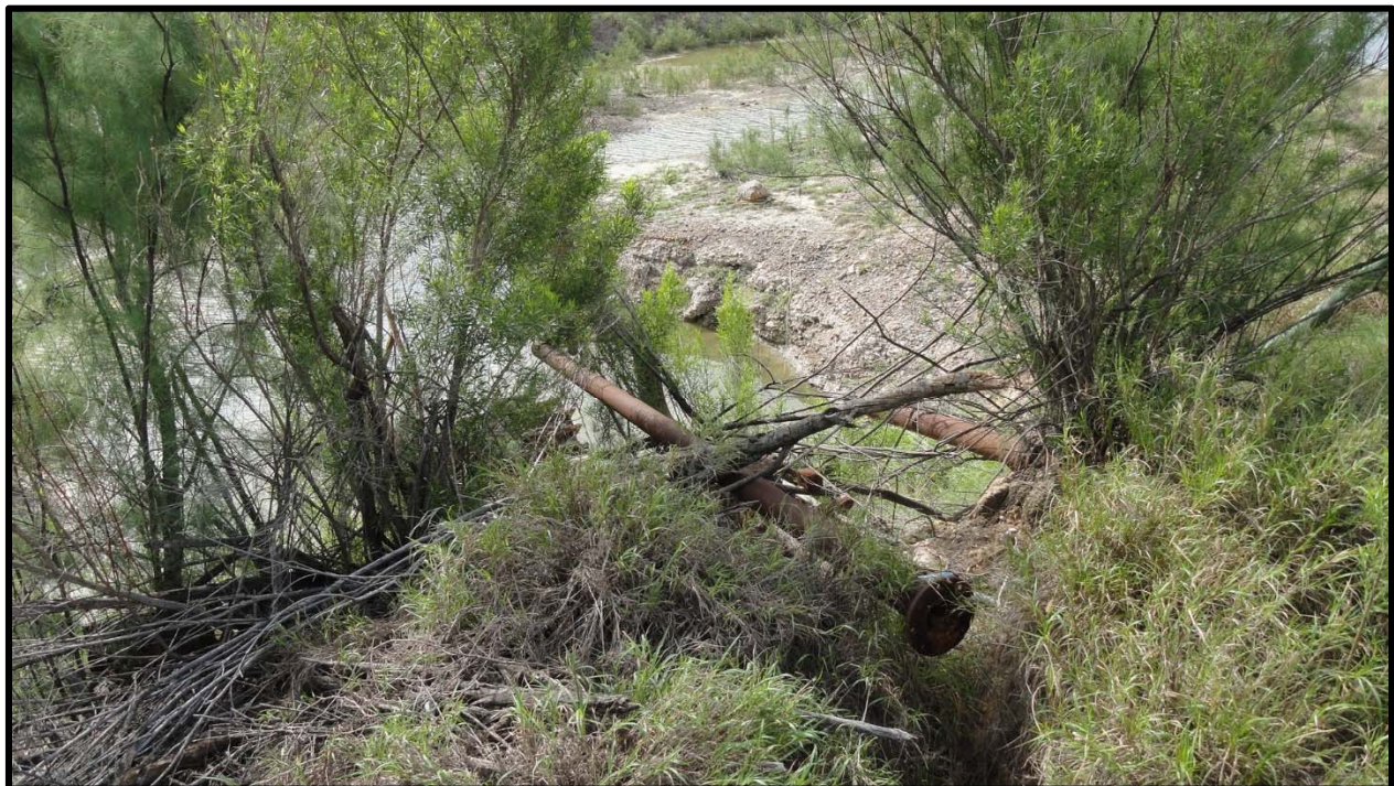
Old metal pump connections at the end of the northeast access road.
