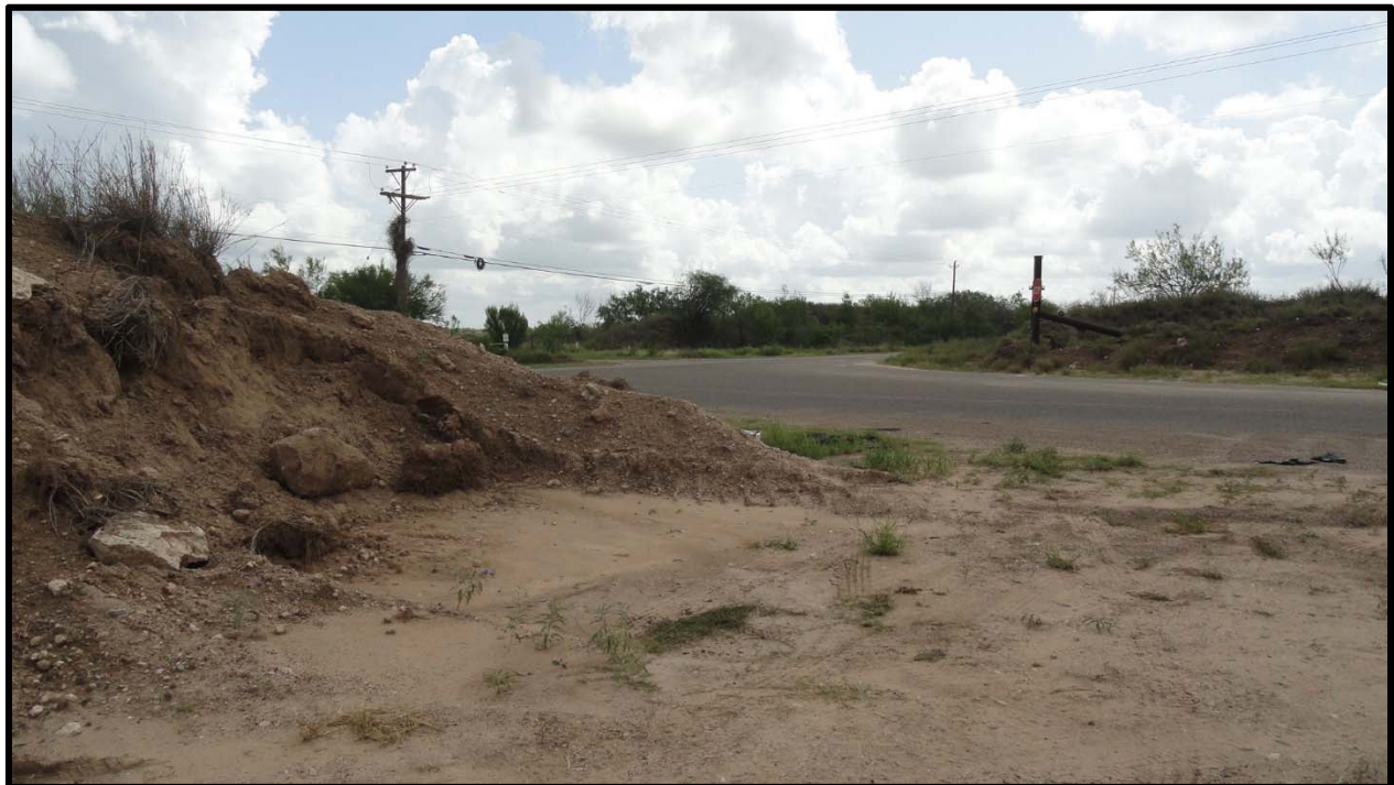
Viewing northeast at Iowa Road and Mile 3 North Road intersection (northeast access road).
