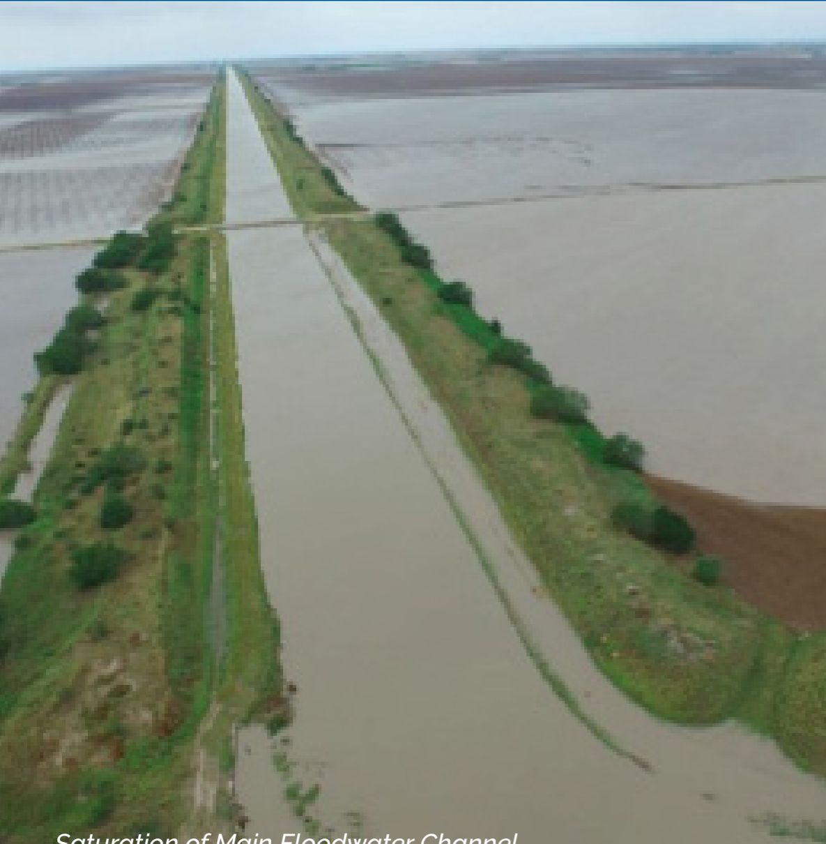
Saturation of Main Floodwater Channel
