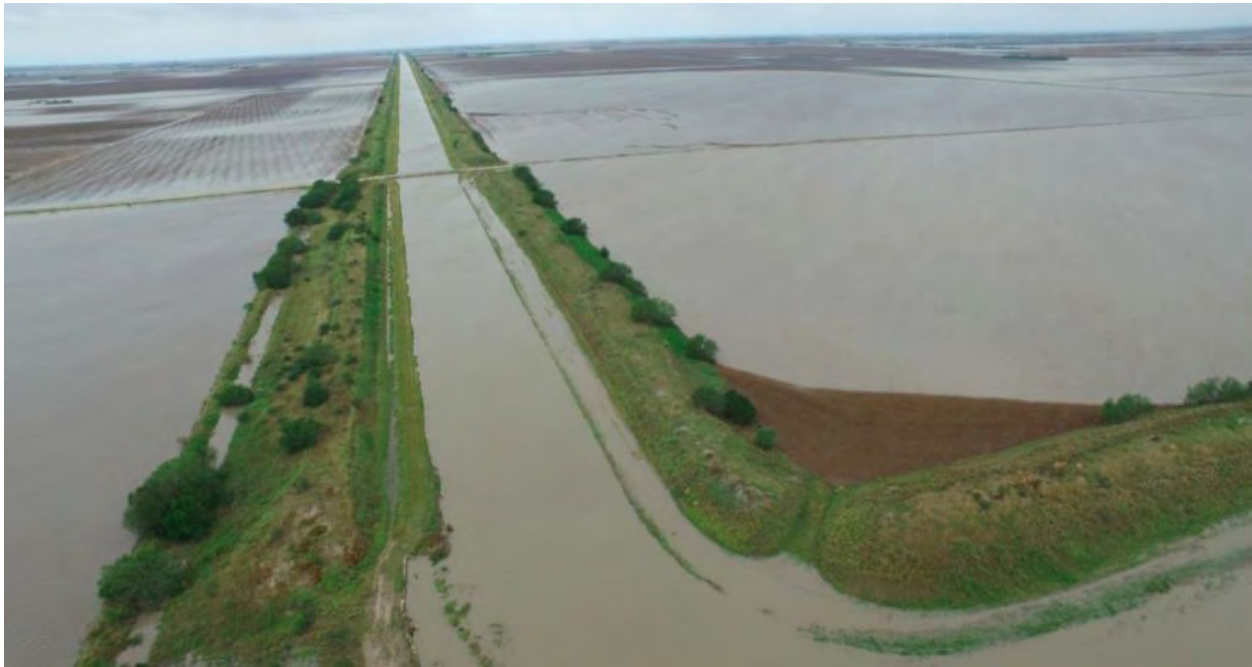
Image Showing Saturation of Main Floodwater Channel During Storm Event
