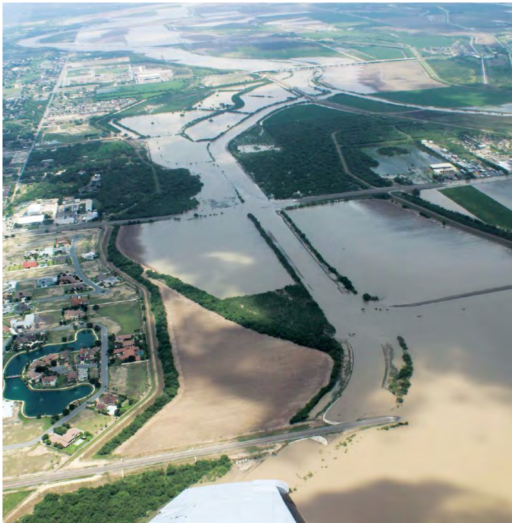
Image Showing Saturation of Drainage Ditch in Hidalgo County
