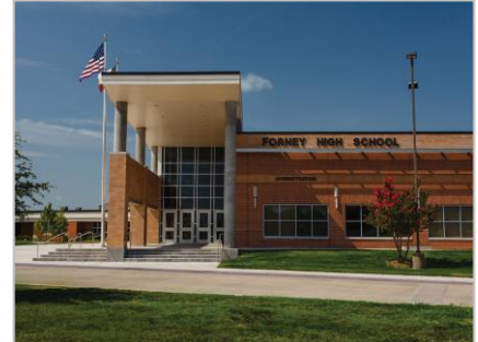
Work at Forney High School includes lighting retrofits, occupancy sensors, and building controls
