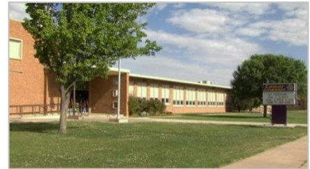
Rooftop DX units were replaced at Lamar Elementary, improving the indoor environment for students and staff.
