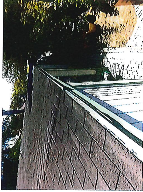
Deteriorated shingles and sagging roof decking
