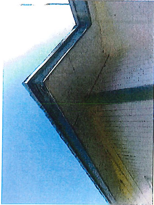
Soffit and Fascia
