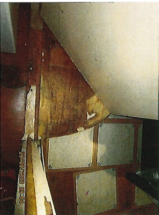
Subfloor rotten away / sunlight through flooring material
