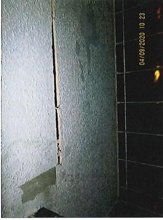
Gypsum boards falling/Tub is leaking
