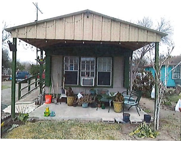
Front of the house facing south
