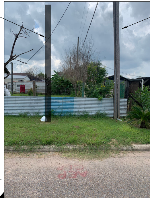
EXISTING POWER POLE
