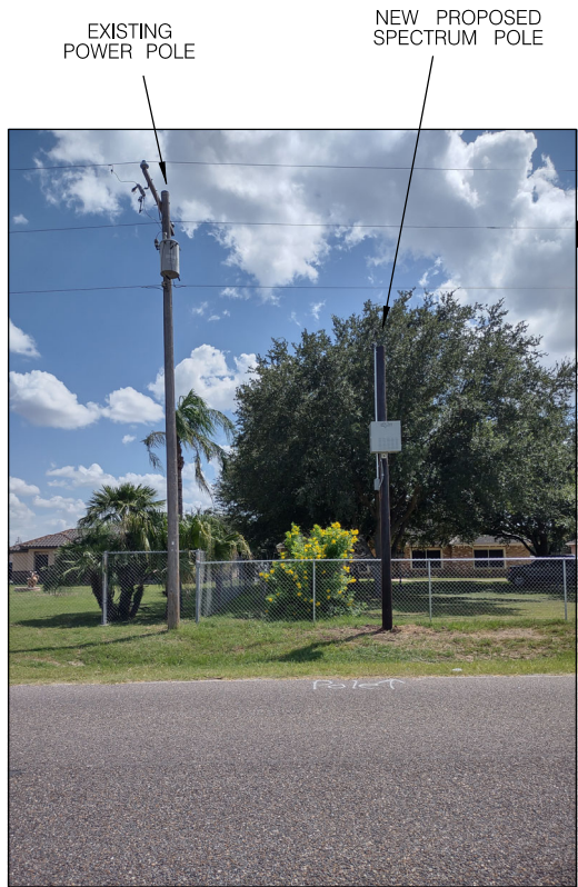
EXISTING POWER POLE NEW PROPOSED SPECTRUM POLE LAT: 26.289029 LONG: -98.119969 NEW PROPOSED SPECTRUM POLE 6' IN ROW & 18' FROM EOP
