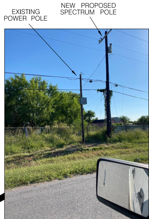
EXISTING POWER POLE NEW PROPOSED SPECTRUM POLE LAT: 26.160843 LONG: -98.096790 NEW PROPOSED SPECTRUM POLE 2' IN ROW & 26' FROM EOP
