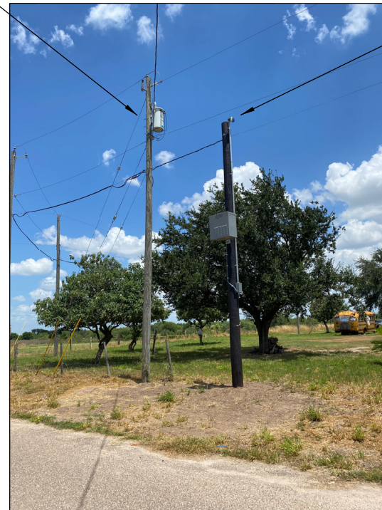
LAT: 26.368045 LONG: -98.007472 NEW PROPOSED SPECTRUM POLE 2' IN ROW & 13' FROM EOP
