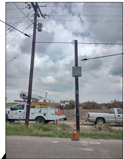
LAT: 26.256352 LONG: -98.073455 NEW PROPOSED SPECTRUM POLE 2' IN ROW & 7' FROM EOP
