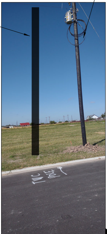
LAT: 26.263060 LONG: -98.065881 NEW PROPOSED SPECTRUM POLE 2' IN ROW & 8' FROM EOP
