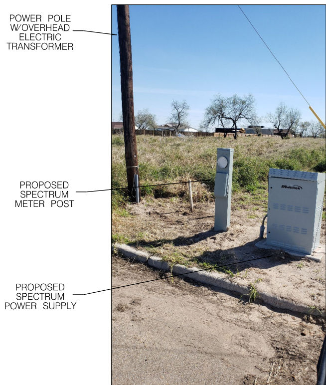
LAT: 26.331157 - LONG: -98.087158 NEW SPECTRUM UG POWER SUPPLY 3' IN ROW & 4.5' FROM EOP
