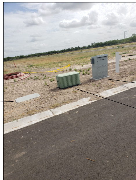
LAT: 26.340705 LONG: -98.102470 NEW SPECTRUM UG POWER SUPPLY 2.5' IN ROW & 5' FROM EOP
