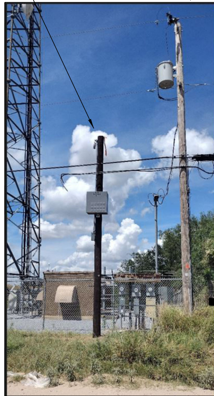
LAT: 26.303249 LONG: -98.387218 NEW PROPOSED SPECTRUM POLE 2' IN ROW & 17' FROM EOP
