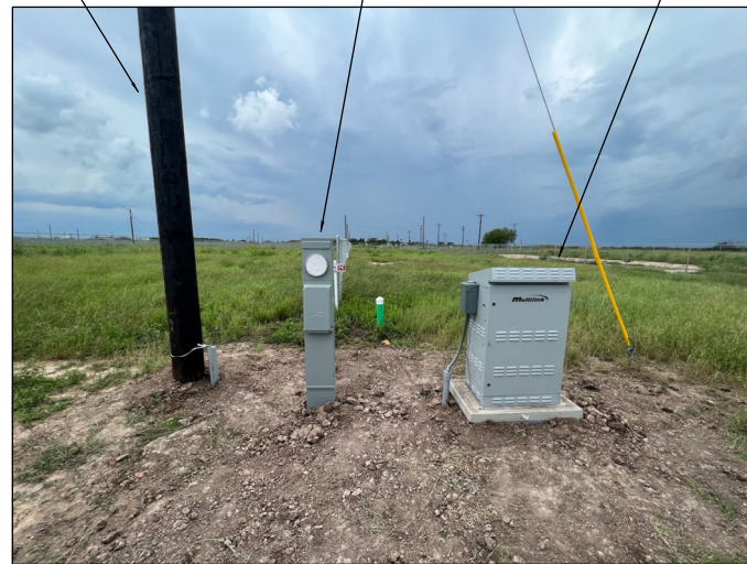
LAT: 26.261587 - LONG: -98.097227 NEW SPECTRUM UG POWER SUPPLY 3' IN ROW & 4.5' FROM EOP
