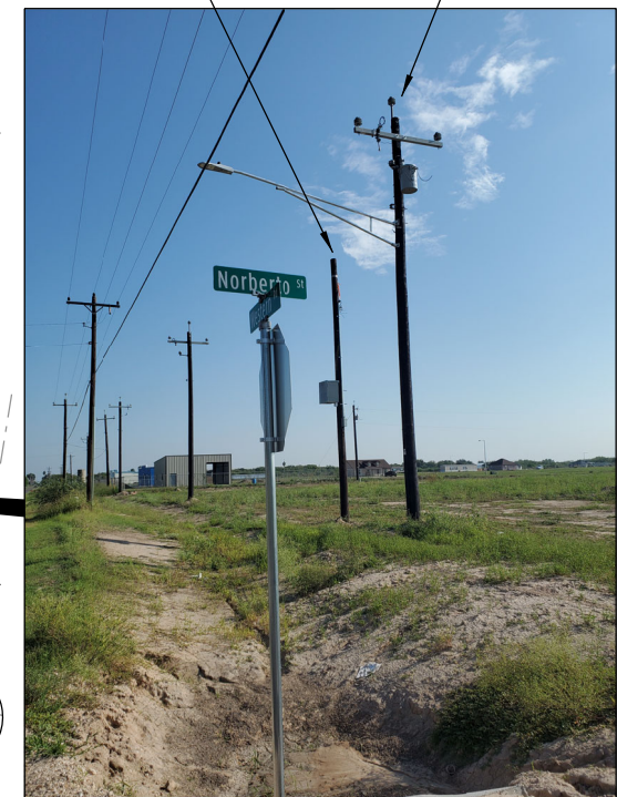
LAT: 26.318102 LONG: -98.393299 NEW PROPOSED SPECTRUM POLE 2' IN ROW & 38' FROM EOP
