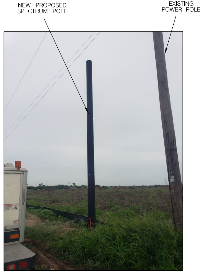
LAT: 26.125774 LONG: -98.043673 NEW PROPOSED SPECTRUM POLE 2' IN ROW & 10' FROM EOP
