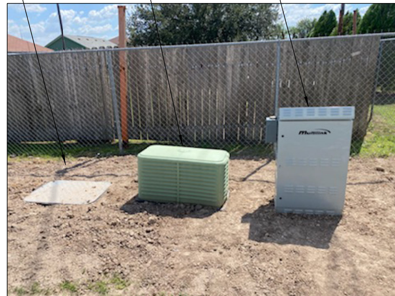
LAT: 26.328339 LONG: -98.070813 NEW SPECTRUM UG POWER SUPPLY 2.5' IN ROW & 5' FROM EOP
