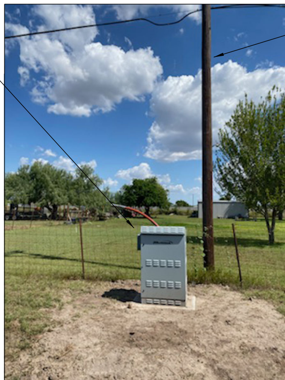
LAT: 26.325601 LONG: -98.067169 NEW SPECTRUM UG POWER SUPPLY 1' IN ROW & 11.5' FROM EOP
