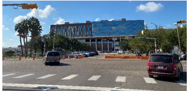
Figure 2 - Existing High-Visibility Crosswalk
