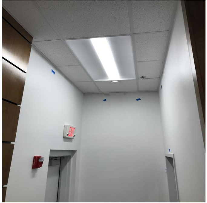
B108 restroom. Grout missing from corners and paint touch up need above frame
