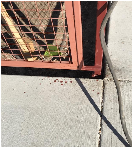
Metal fence needs to be painted and primer removed from sidewalks
