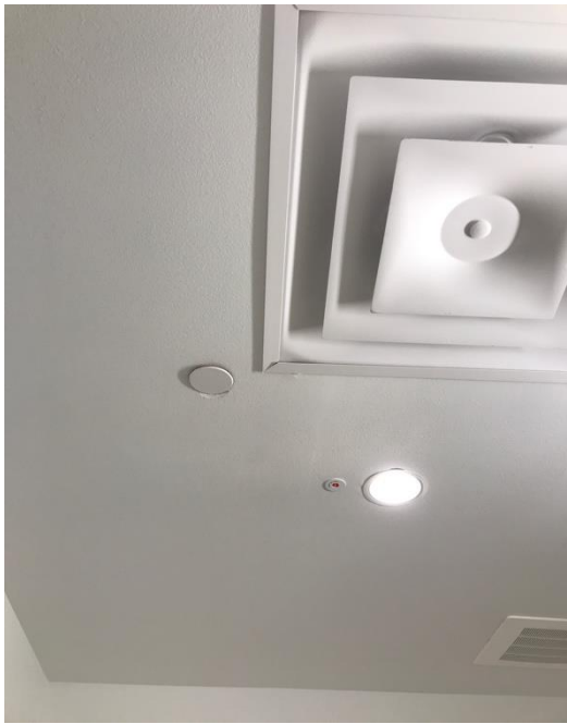
Escutcheons missing and both men's and women's restrooms. Texture and paint touch ups needs around air vents
