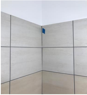
B108 restroom. Grout missing from corners and paint touch up need above frame
