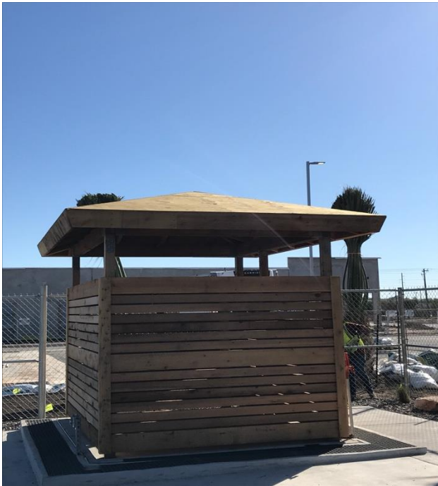
Shingles missing from kennel
