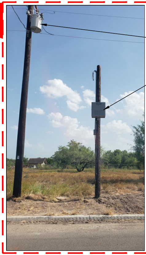
LAT: 26.308649° - LONG: -98.552481° NEW SPECTRUM POLE MOUNTED POWER SUPPLY 2' NORTH FROM ROW & 7' SOUTH FROM EOP
