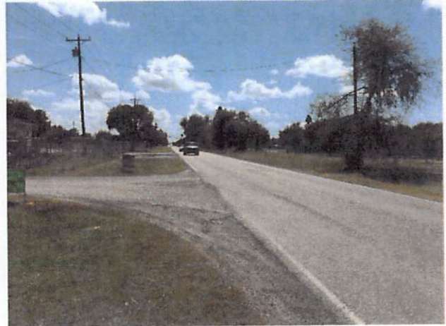
Photo 2 Southern view of Cesar Chavez Road
