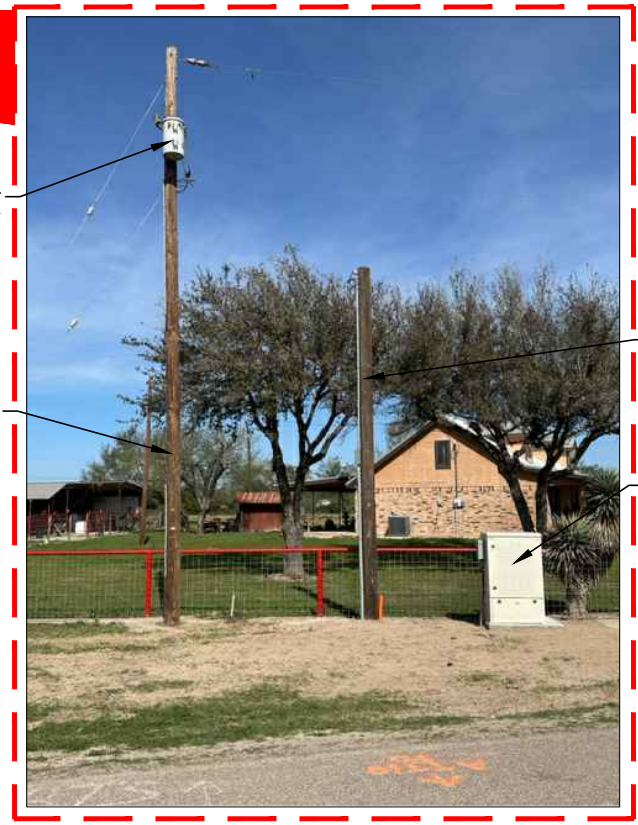
LAT: 26.348715° - LONG: -98.181919° NEW SPECTRUM UNDERGROUND POWER SUPPLY 2' SOUTH FROM ROW & 18' NORTH FROM EOP
