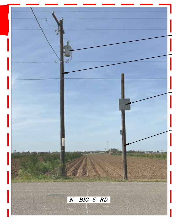
LAT: 26.355029° - LONG: -98.196743° NEW SPECTRUM POLE MOUNTED POWER SUPPLY 1' EAST FROM ROW & 8' WEST FROM EOP
