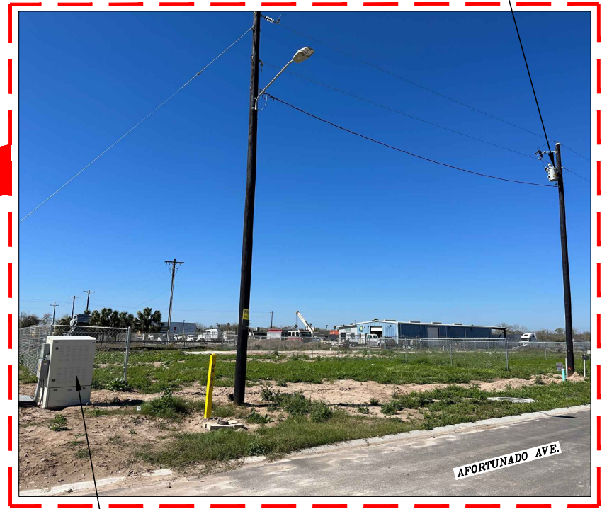
A.E.P. POLE & TRANSFORMER SPECTRUM POWER SUPPLY UNIT LAT 26.1 73 6 - LONG -9 .063670 NEW SPECTRUM UNDERGROUND POWER SUPPLY 2' EAST FROM ROW & 10' WEST FROM EOP
