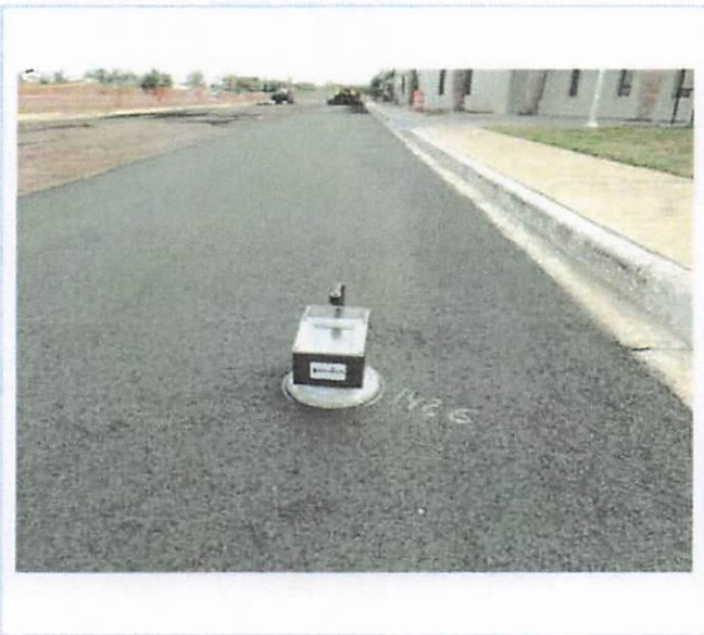
(P2) NW driveway 2.5 thickness.
