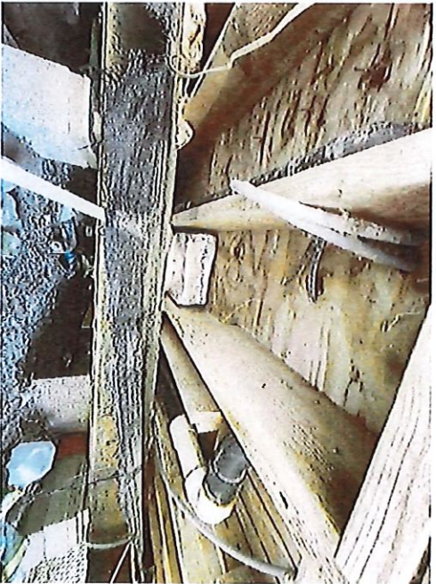
sewer lines not properly supported
