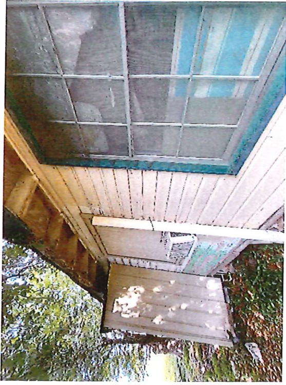
Soffit and Fascia
