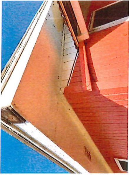
Soffit and Fascia
