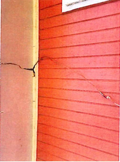
Exposed electrical wires
