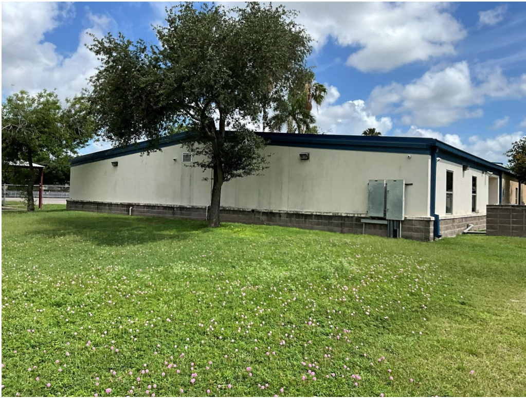
Southern Elevation of Wing A
