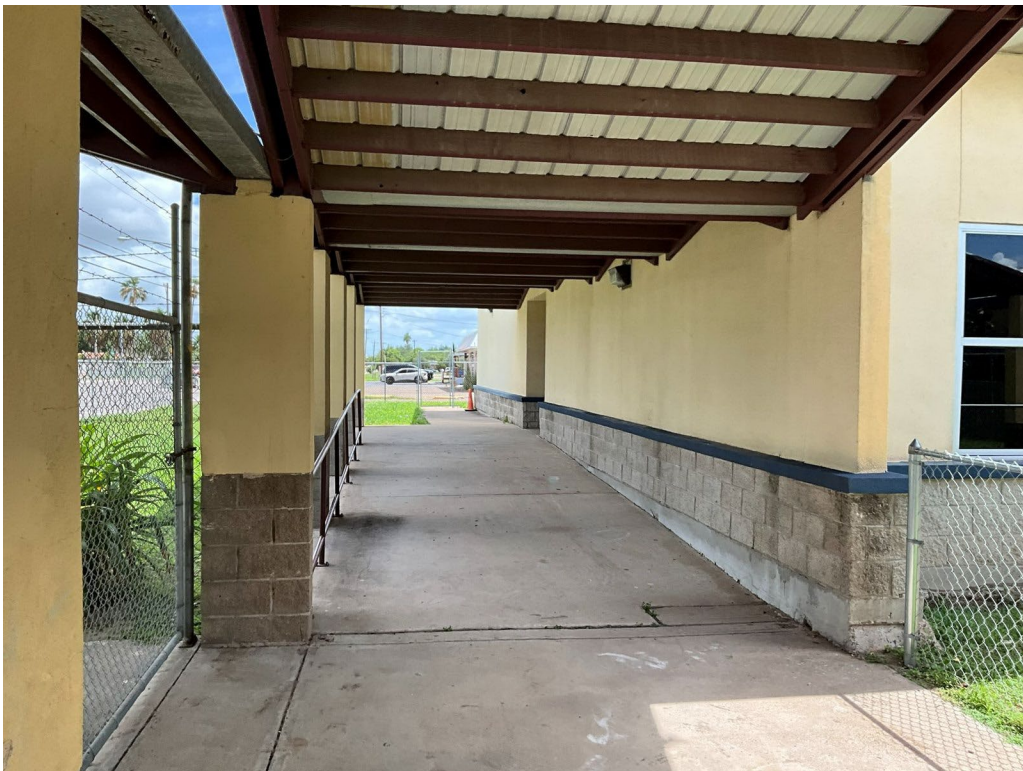
Western Elevation of Wing B
