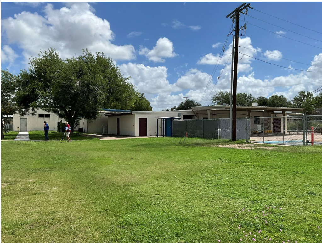
Southern Elevation of Library / Storage / Kitchen
