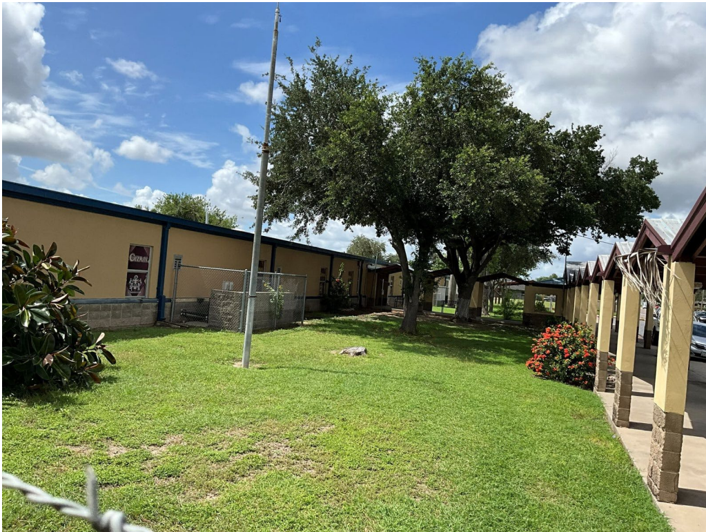
Western Elevation of Wing A
