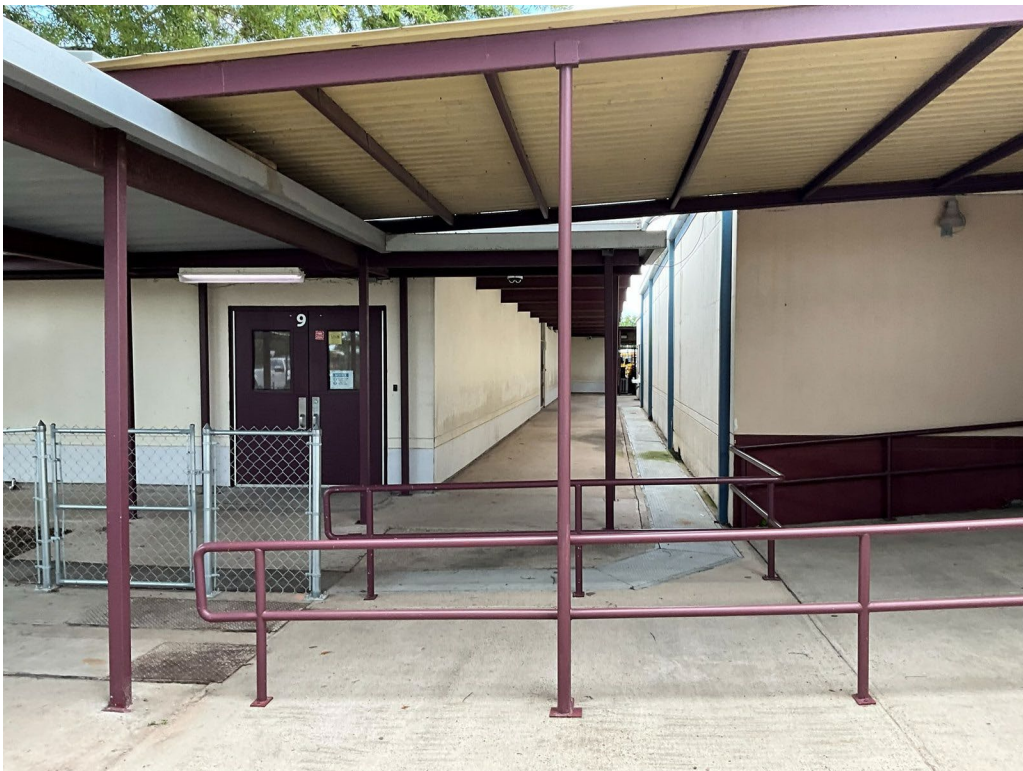
Covered walkway between library and kitchen facing south
