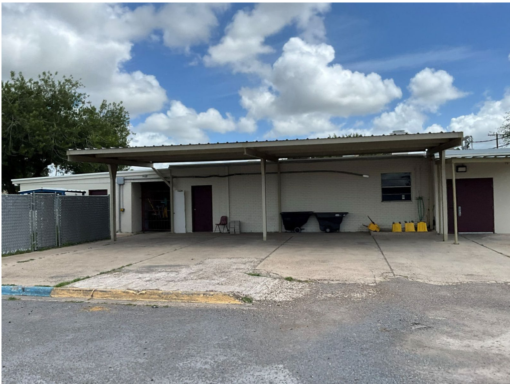
Southern Elevation of Storage Building and Kitchen Facility
