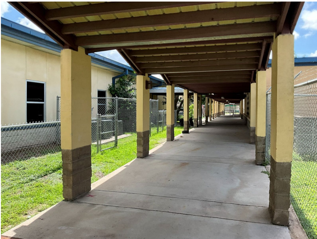
Walkway between Wing B, Wing A, & Teacher Work Area / Lounge / Clinic
