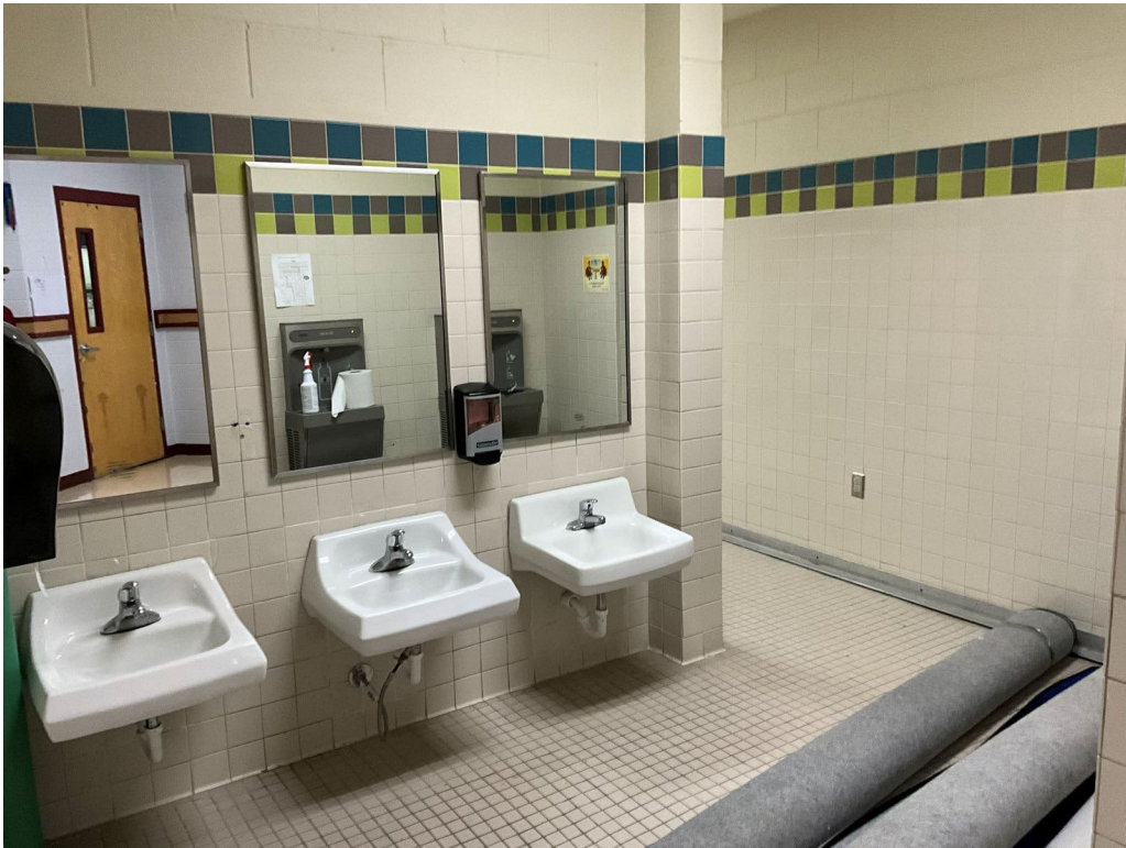
Restroom in Wing B
