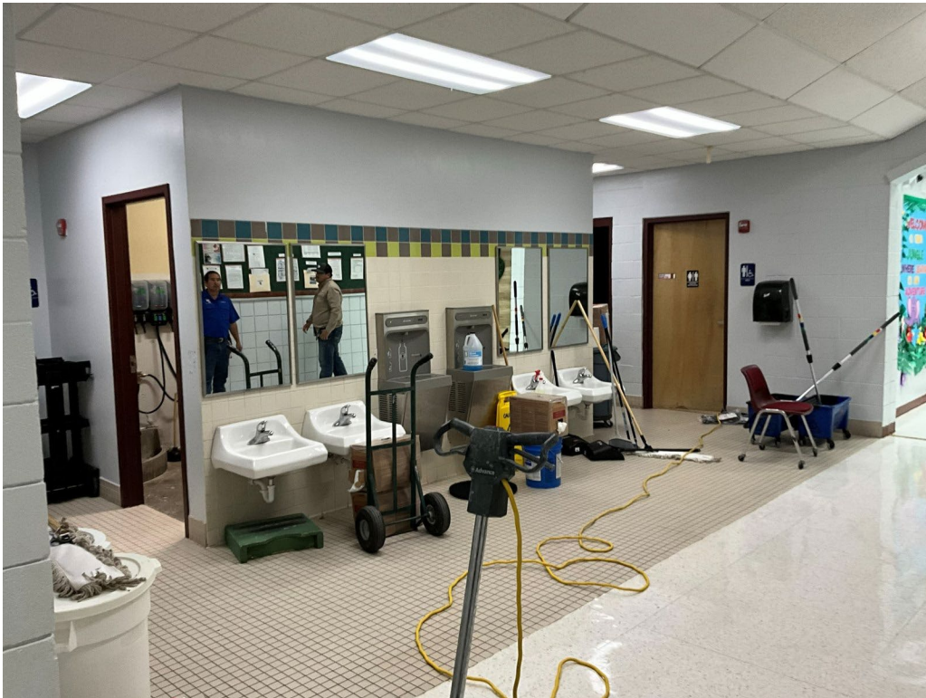
Restroom entry area and water closet in Wing A
