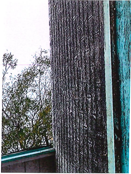
Roof Soffit and Fascia
