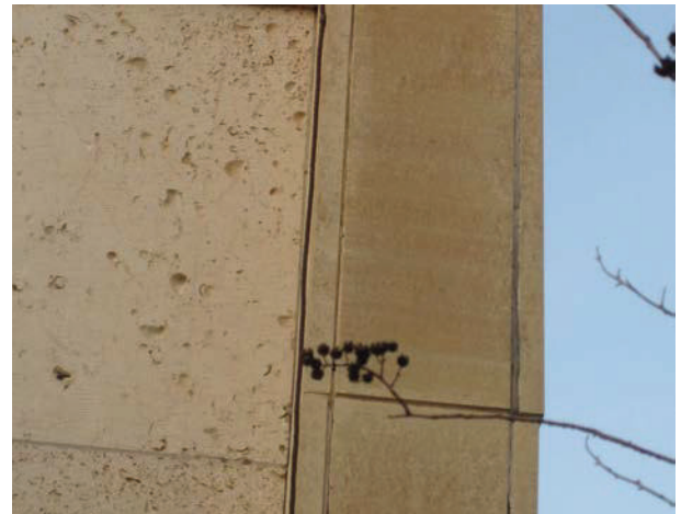
Some of the dolomitic limestone panels have been re-attached with surface mounted fasteners, such as the unit at the far right.
