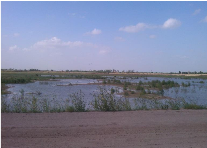
Photo 3 View of detention pond in use.
