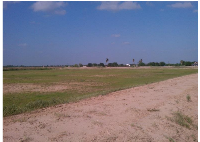
Photo 4 View of detention pond
