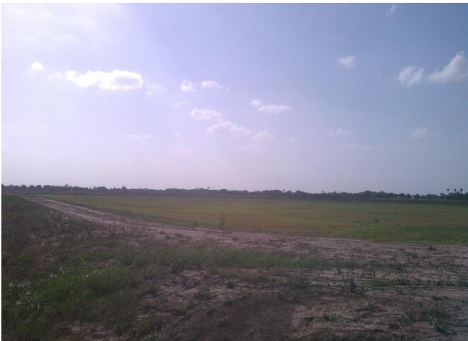
Photo 3 View of Detention Pond
