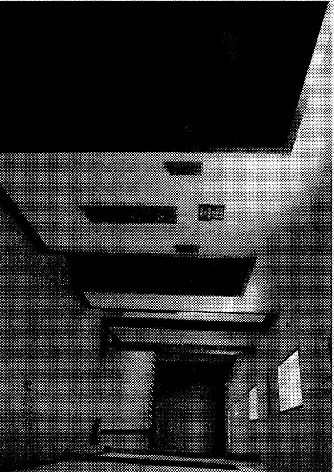
Elevator Lobby 1 st Floor Completed.
