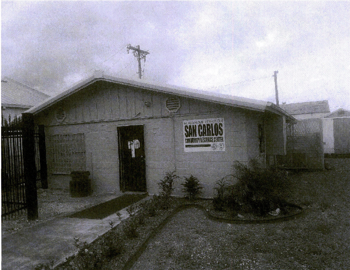
San Carlos Warehouse Bldg# 3 - ID# 3147 | 230 N. 86 th Street, San Carlos, TX 78539
