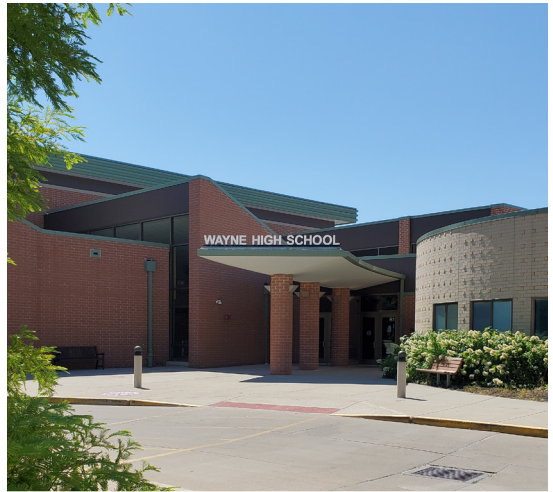
Wayne High School (new complex)
