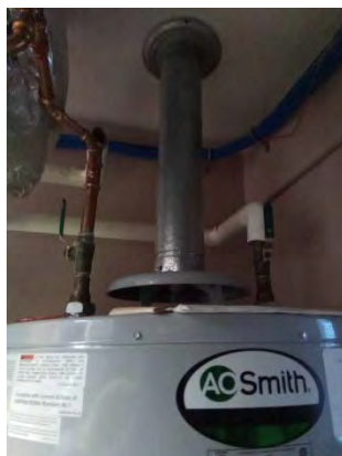
Fire Station 23- Gas Water Heater 100 gallon
