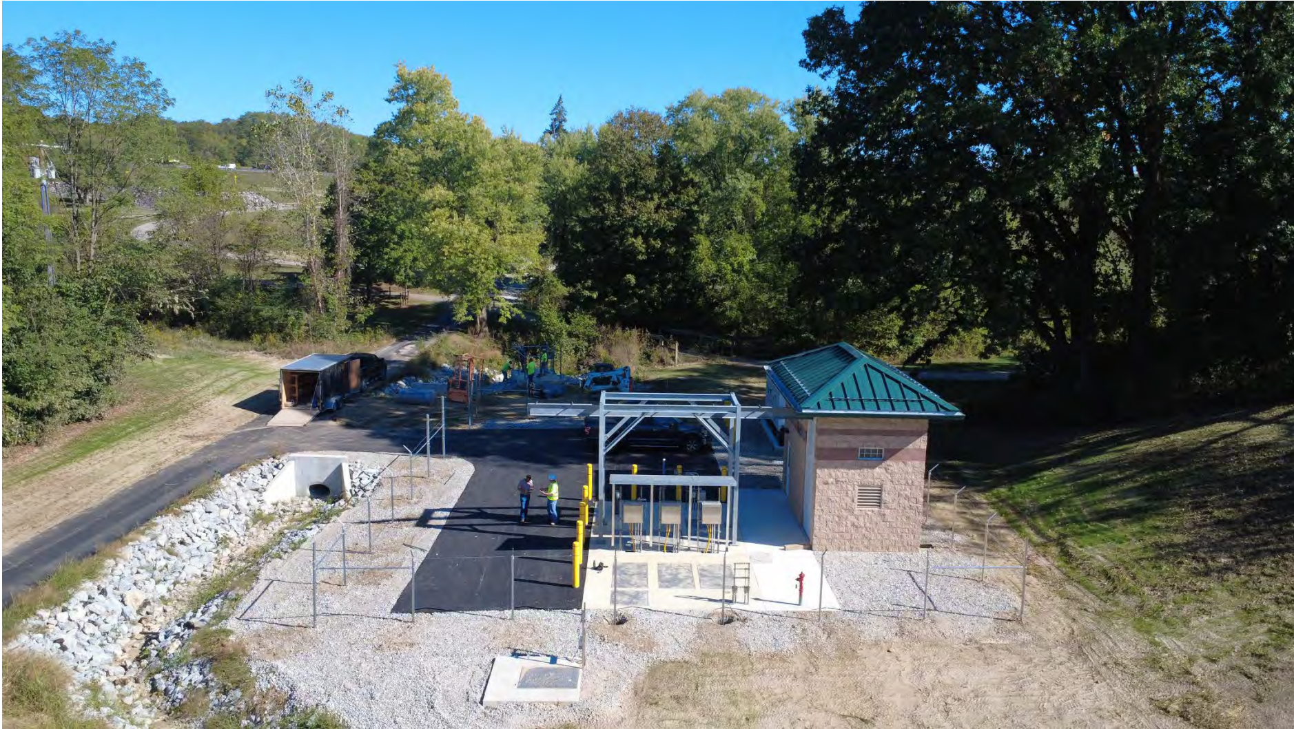
EQ Pump Station/ Diversion Chamber/ Electrical Building – Sept. 2025
