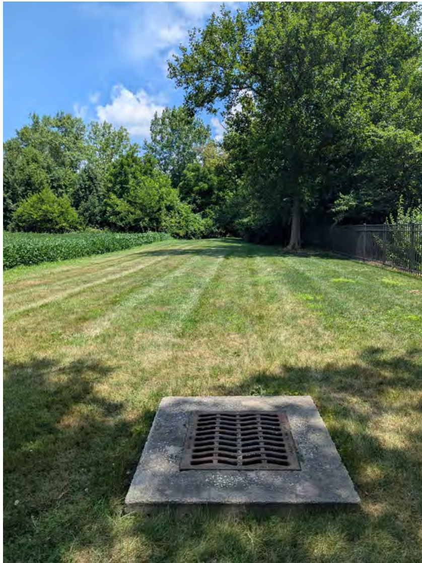
Concrete drainage access structure (catch basin) located near the rear property line of 2591 Blueflag St., facing toward the adjoining farmland/development parcel. Photographed July 12, 2026.
