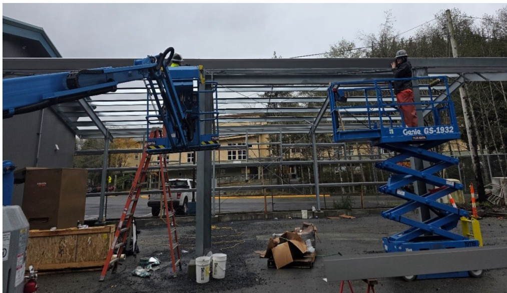
Dawson staff installing the metal frame structure of the roof.
