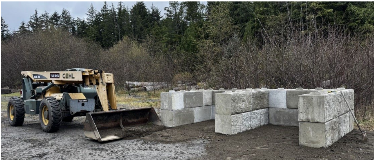
Newly constructed composting area at D-1 property
