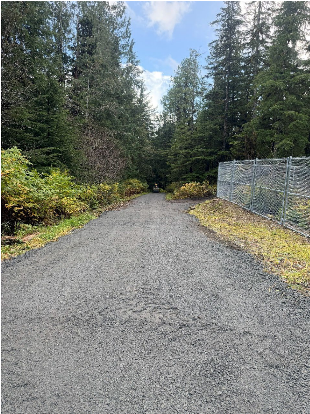
Resurfaced access road to Roosevelt Water Treatment Plant
