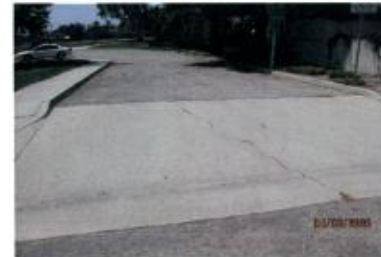
Driveway Approach (Before)
