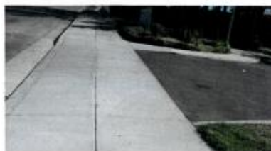
Driveway Approach (After)
