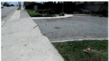
Driveway Approach (Before)
