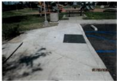
ADA Ramp (After)
