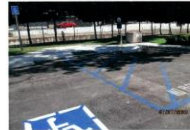
ADA Ramp (After)
