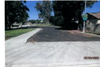
Driveway Approach (After)
